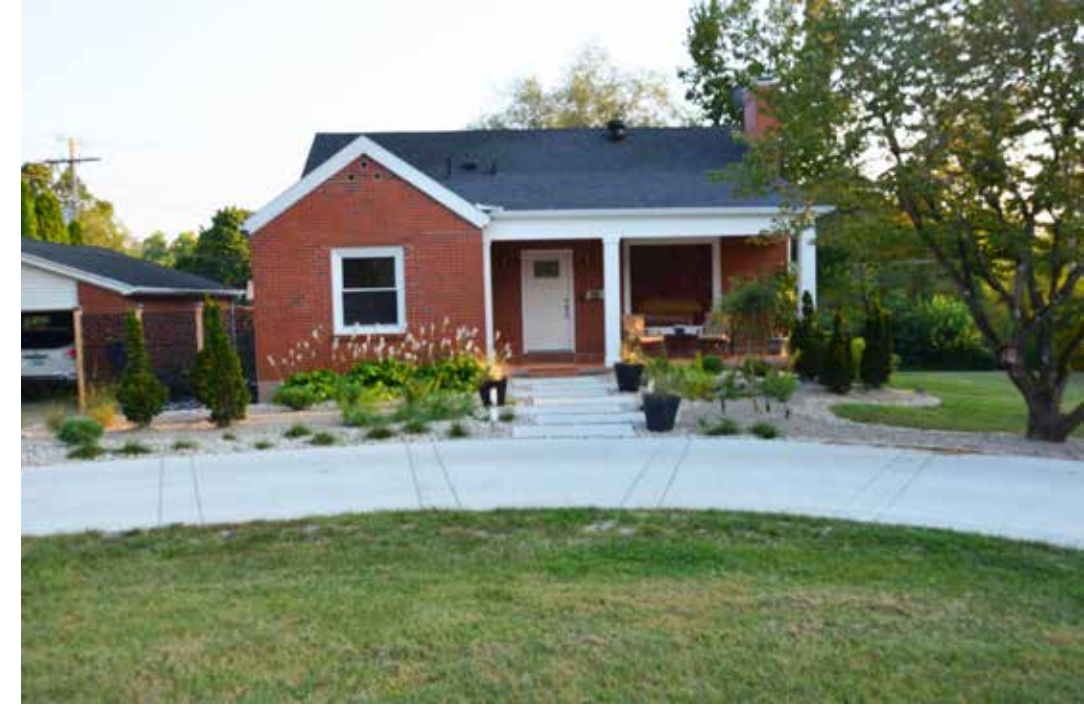
The tiny 4x4-inch columns were replaced by beefy 10-inch columns to complete the look and bring the porch to scale. The traditional dentil fascia board was replaced with a plain board for a cleaner look (right).
